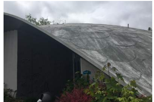
CURRENT ROOF CONDITION
