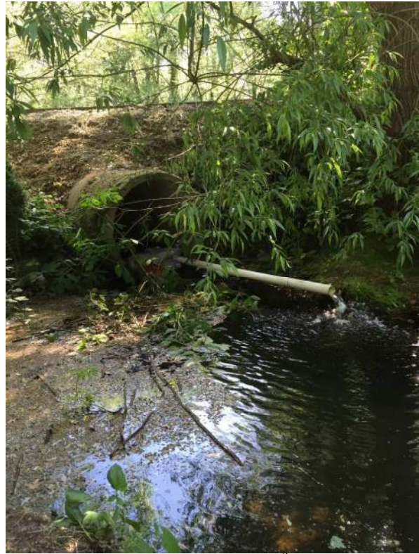
6. Outlet of 4' culvert under 16 th Ave South
