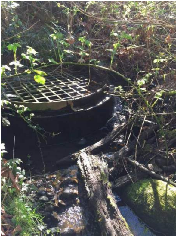
5. Energy dissipater at bottom of hill
