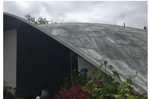
CURRENT ROOF CONDITION
