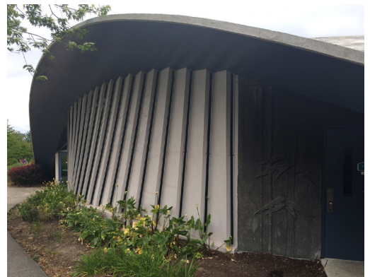
UNDERHANGS AND DOORS TO BE PAINTED
