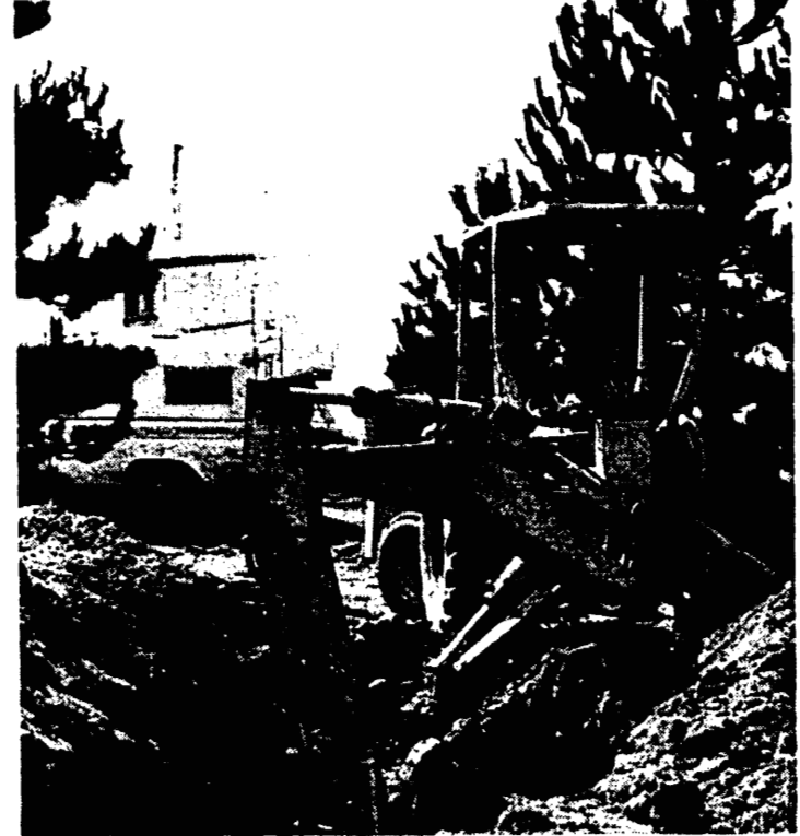
BREAKING GROUND. . . Work has begun on the Phase III construction project to enlarge the campus to meet the growing needs of higher education here.
