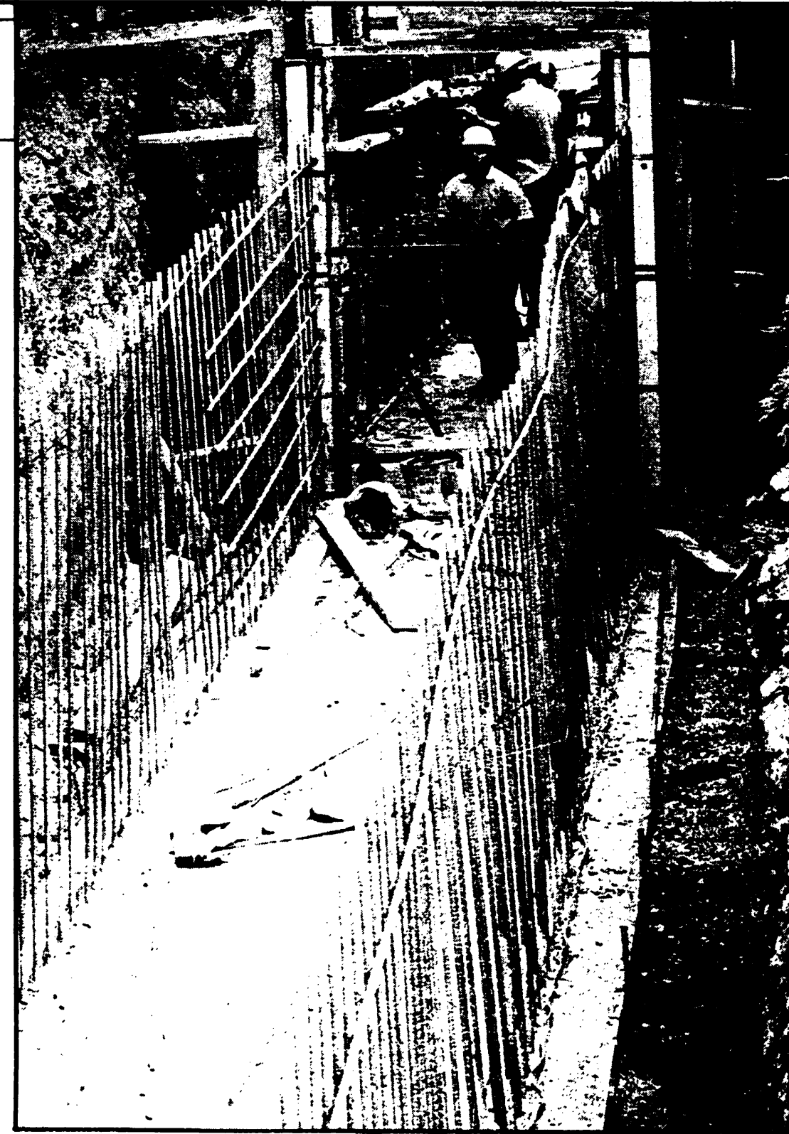
DOWN IN THE TRENCHES ... Workmen place molding over reinforcing rod in a trench. Concrete will be poured over the molding and the reinforcing rod, creating a virtual tunnel which will protect the new heating lines from corrosion and allow easier replacement.
