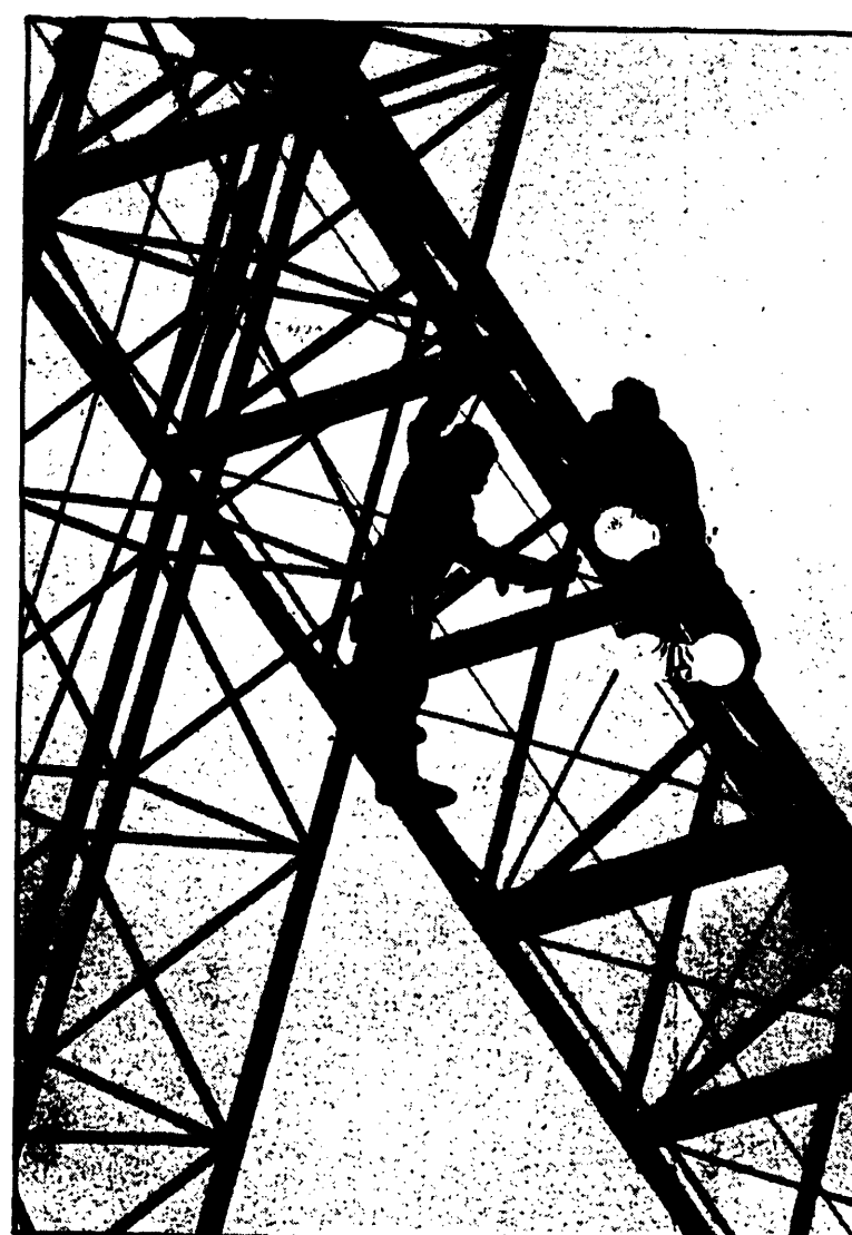
Construction workers edge out toward the end of the boom, six stories off the ground. These two workers connected the second crane to the library crane's boom.
