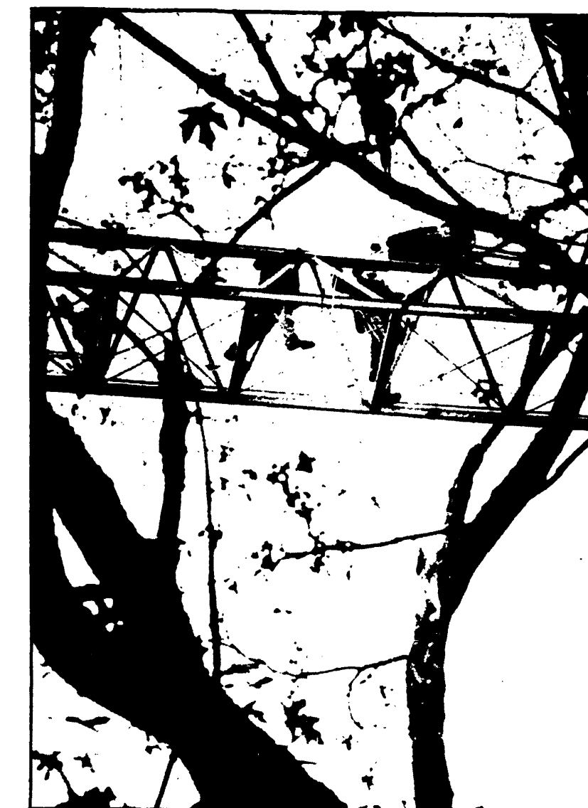
Framed by a near leafless tree, scaffolders connect the second crane's hook to the boom to ready for the lowering operation.
