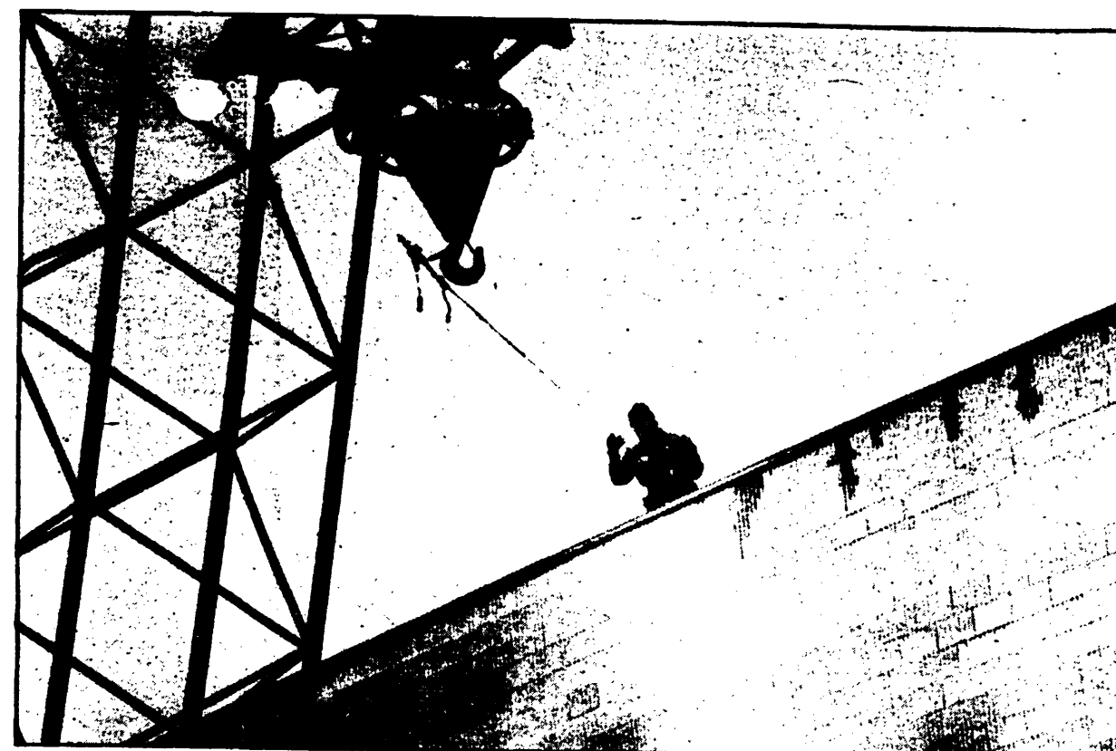
The hook of the crane boom came down first while workers controlled the landing position from the roof and on ground.
