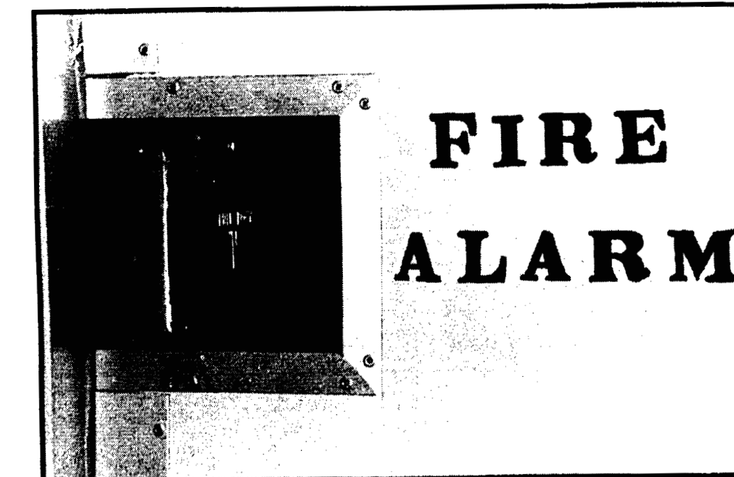
One of the fire alarm pull boxes (pictured above) in building 23 must be accessed by reaching through a hole in the wall.
