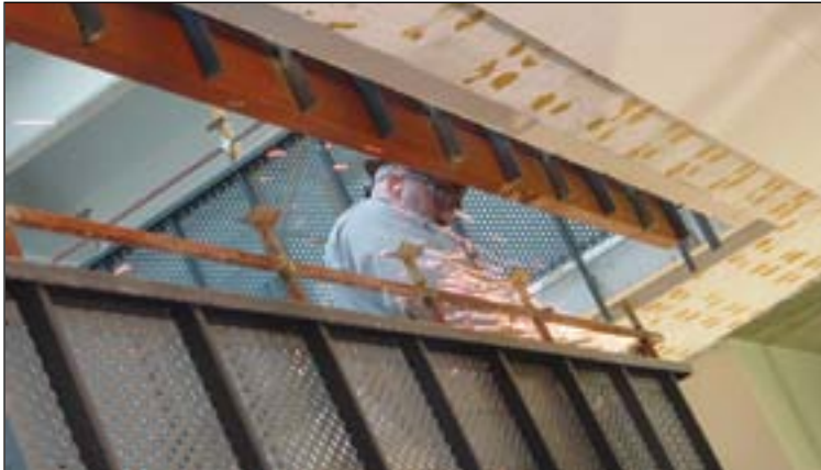
Alisa Gramann/ THUNDERWORD Construction workers grind off rough spots on railing inside Building 9 recently. The remodeling project should be done in mid-February.
