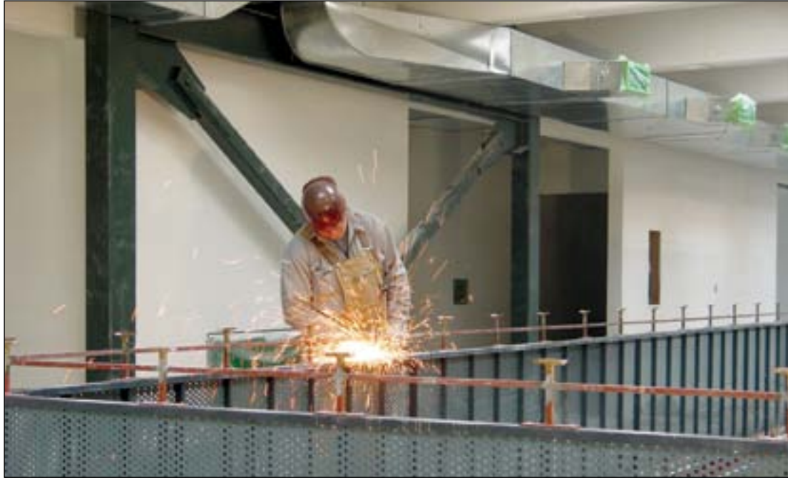
Alisa Gramann/ THUNDERWORD Construction workers grind off rough spots on railing inside Building 9 recently. The remodeling project should be done in mid-February.
