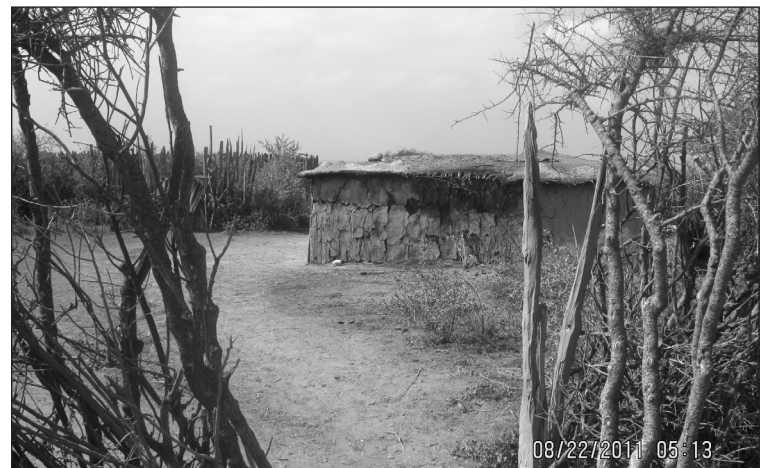
A "boma," a traditional Kanyan house, is made from manure, mud, and sticks.
